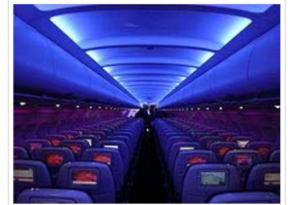
LED lighting in a aircraft cabin of the Airbus A320 Enhanced.
